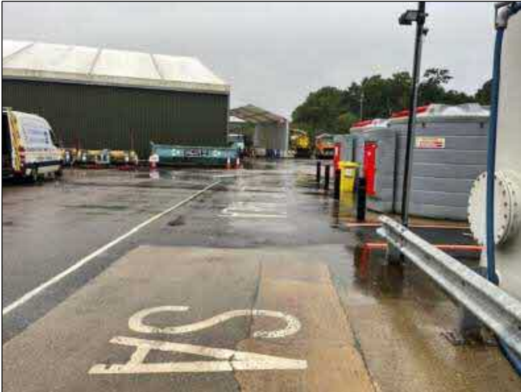
Salt Saturator and Fuel tanks
