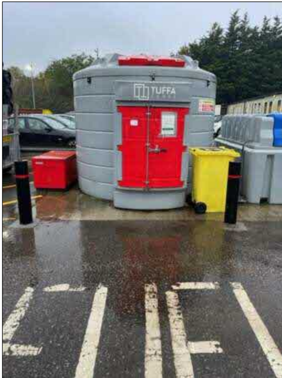
Above ground fuel tanks and fueling area
