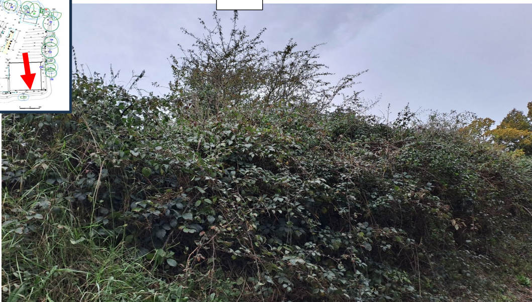
Photo 6 of a general view of the southern bund looking towards G18
