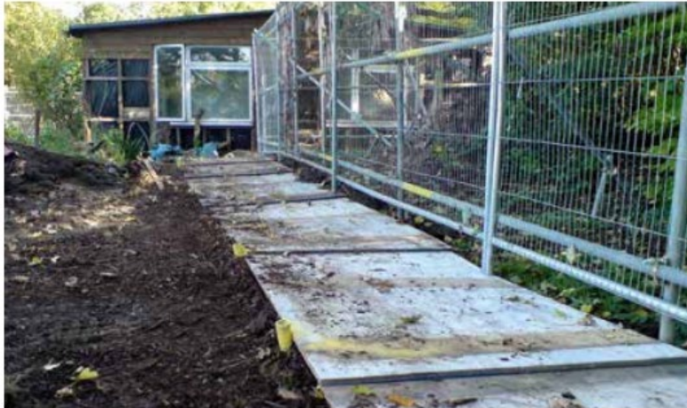
SGN 3-02 Heavy-duty plywood set onto a compressible woodchip layer and pinned into position is suitable to spread the loading from pedestrian access.
