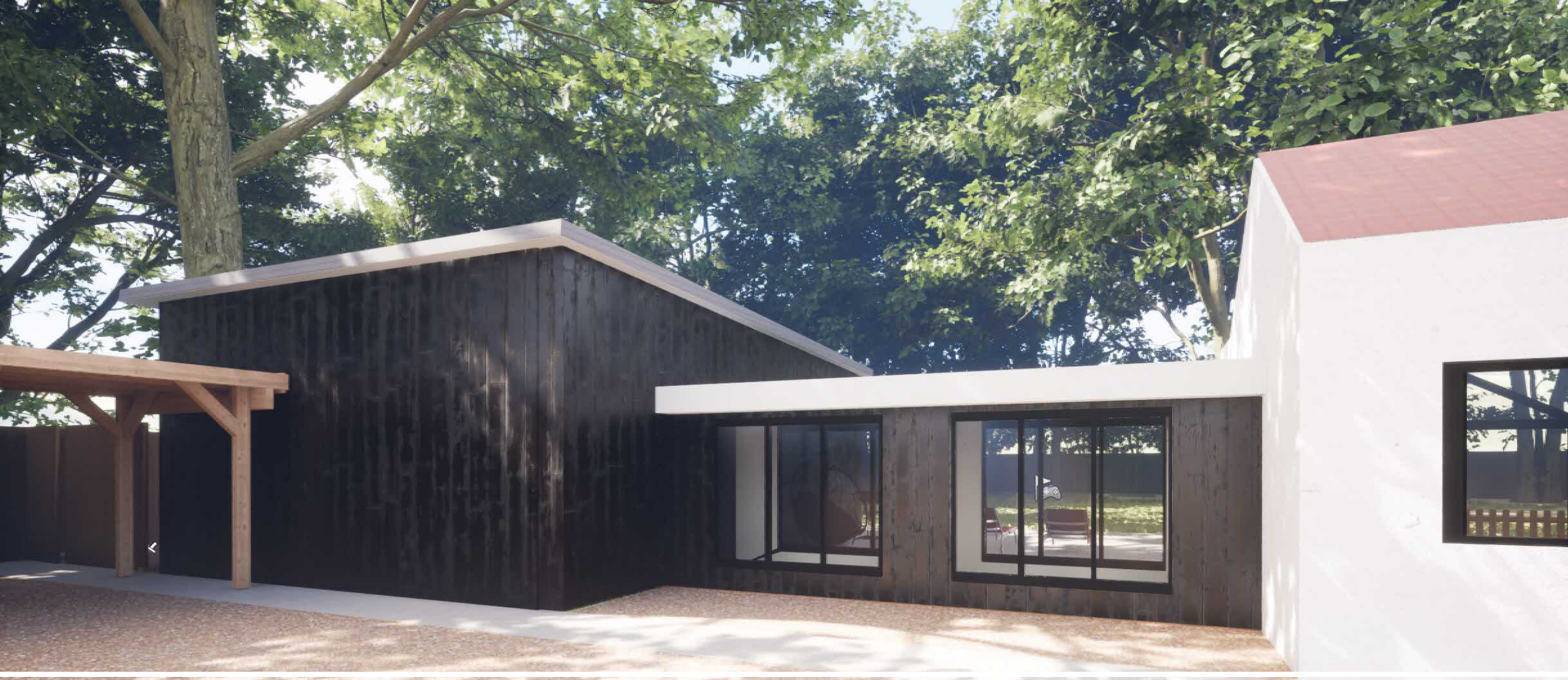
Up close to extension – dark wood clad glass hallway transparently connecting cottage
