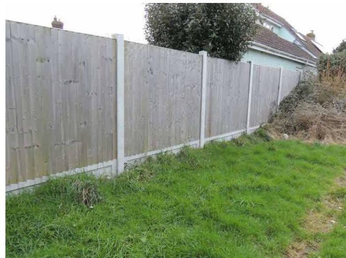
Photo 9: Looking southwards along eastern boundary. The small pile of brush is to be cleared by hand
