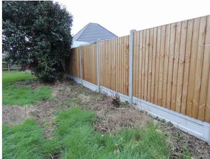
Photo 4: Looking southwards along western boundary
