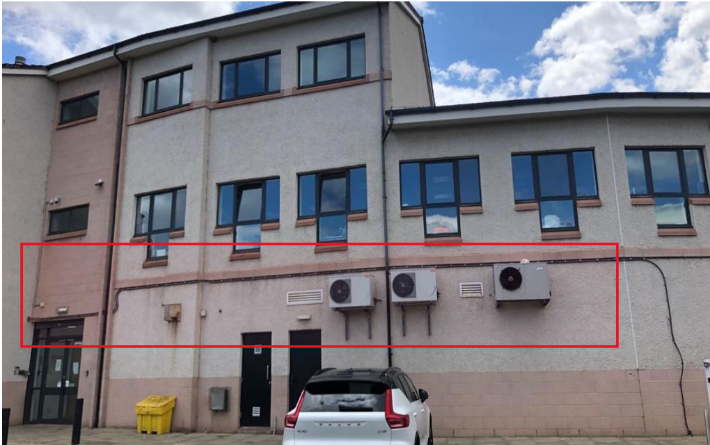
Existing M&E and extract grills to rear of building
