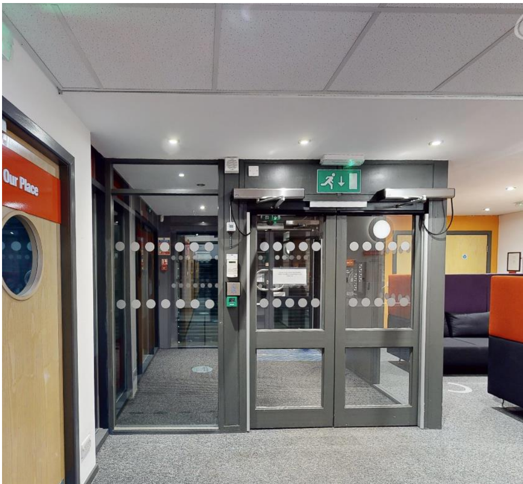
Existing Draft/Security lobby.
