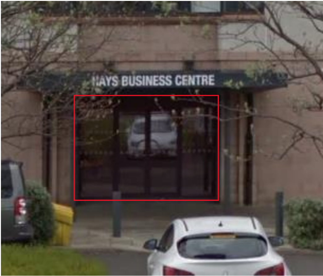
Existing entrance doors [location of proposed sliding doors]
