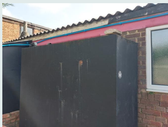
Above-ground heating oil tank on site beneath corrugated cement roofing contain potential
