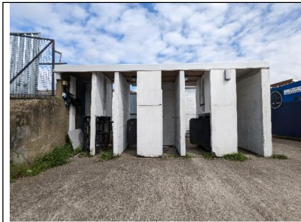
Photograph 15: Southern elevation of Building 6
