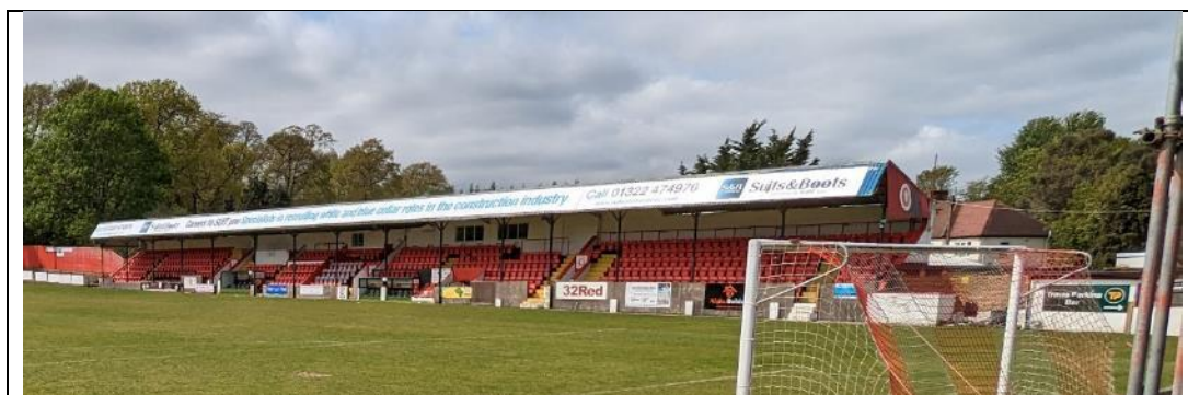
Photograph 12: Eastern elevation of Buildings 3 and 4
