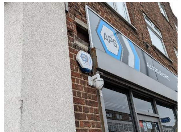
Photograph 9: Cavity formed by I-beam on Building 1
