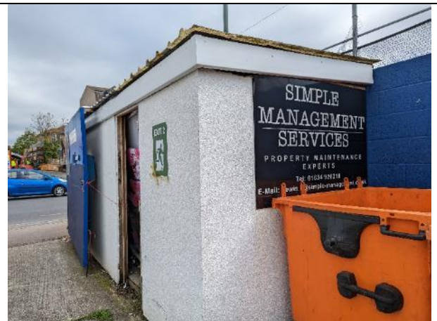
Photograph 16: Southern and western elevations of Building 7
