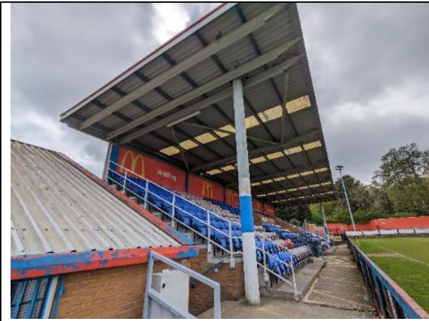
Photograph 19: Western elevation of Building 10
