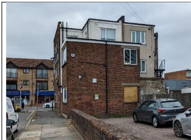
Photograph 10: Southern elevation of Building 2
