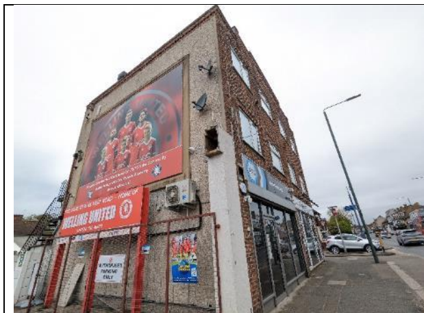
Photograph 8: Northern and eastern elevations of Building 1
