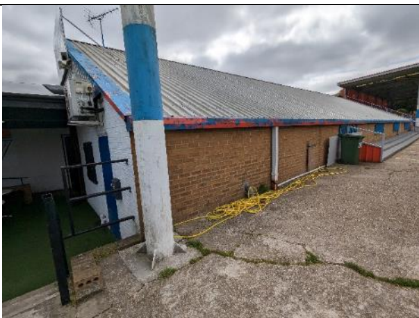
Photograph 18: Northern and western elevations of Building 9
