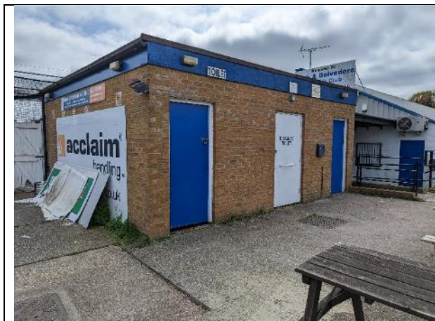
Photograph 17: Northern and western elevations of Building 8
