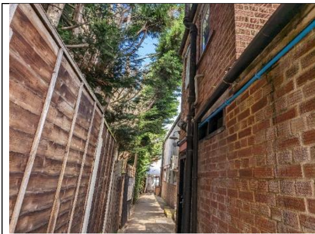
Photograph 13: Western elevation of Building 5
