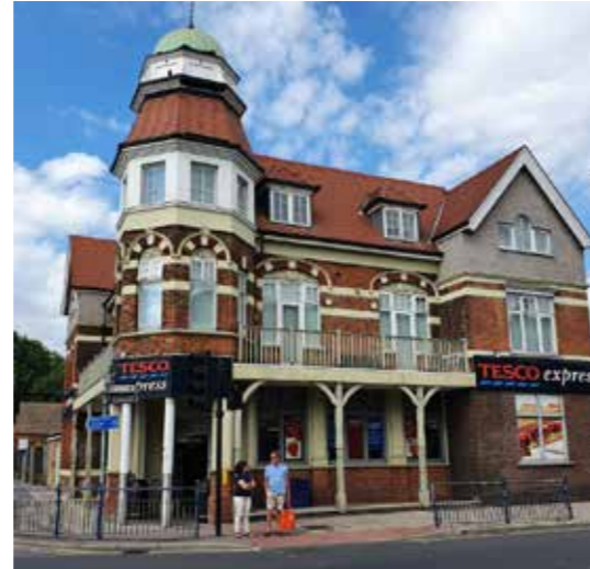
Tesco (formerly The Station Inn) -locally listed
