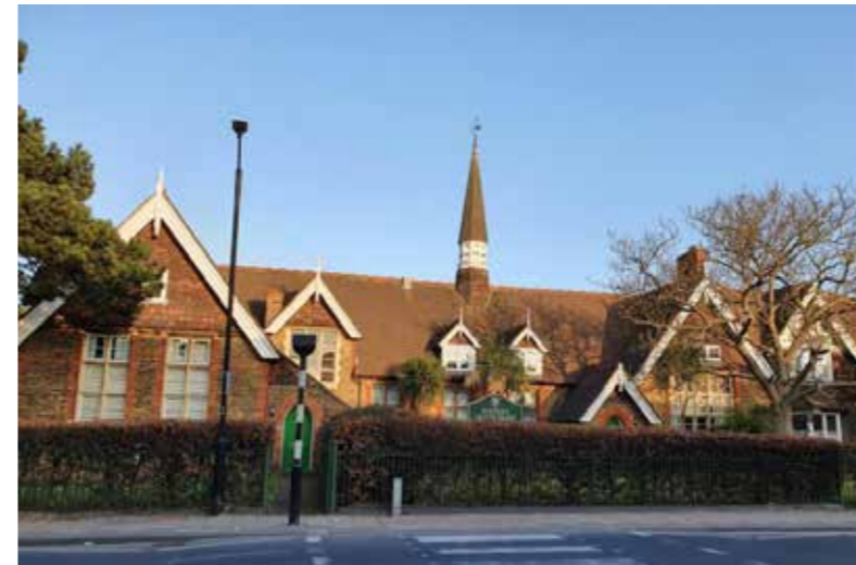
Former Fosters Primary School - Grade II listed
