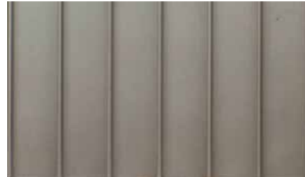
Standing seam aluminium roofing
