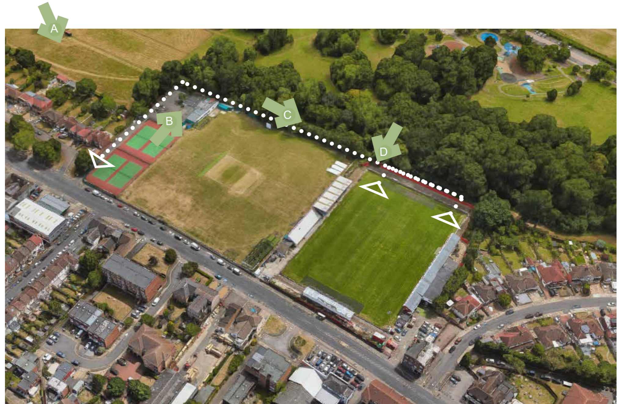
AERIAL VIEW INDICATING EMERGENCY EGRESS FROM EXITS C & D THROUGH DANSON PARK
