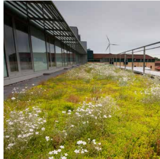
INTENSIVE GREEN ROOFS
