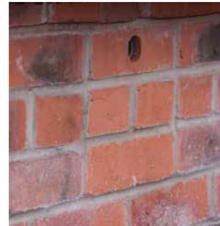
Built in starling boxes designed to fit within brick dimensions. Woodstone invisible box
