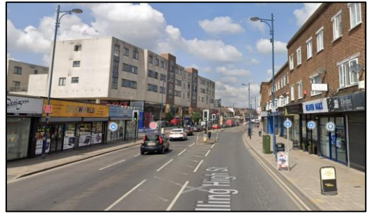
Embassy Court, Welling Town Centre
