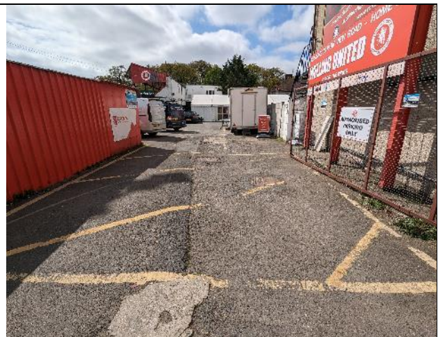
Photograph 4: Buildings and hardstanding in the north-west of the site
