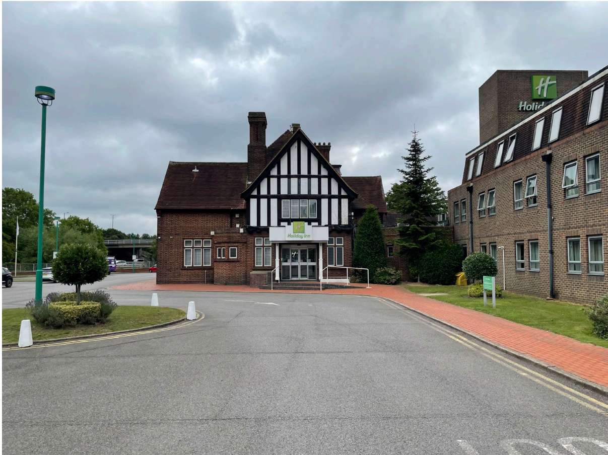
View of current entrance to the hotel
