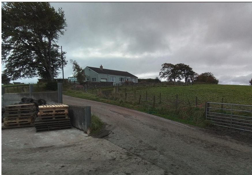
Fig 6 -View of the dwelling to the south
