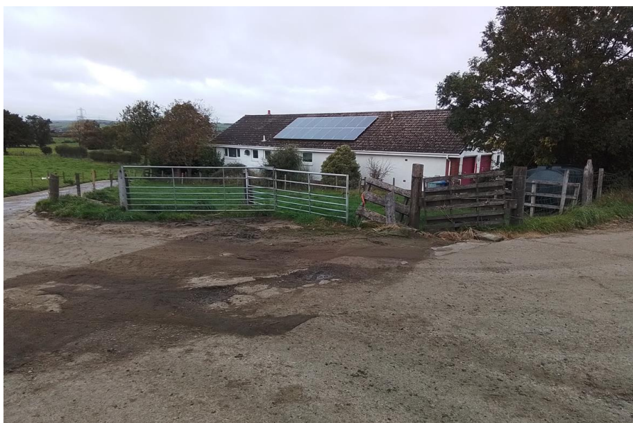
Fig 2 -View of the dwelling to the north adjacent to the existing farm access-
