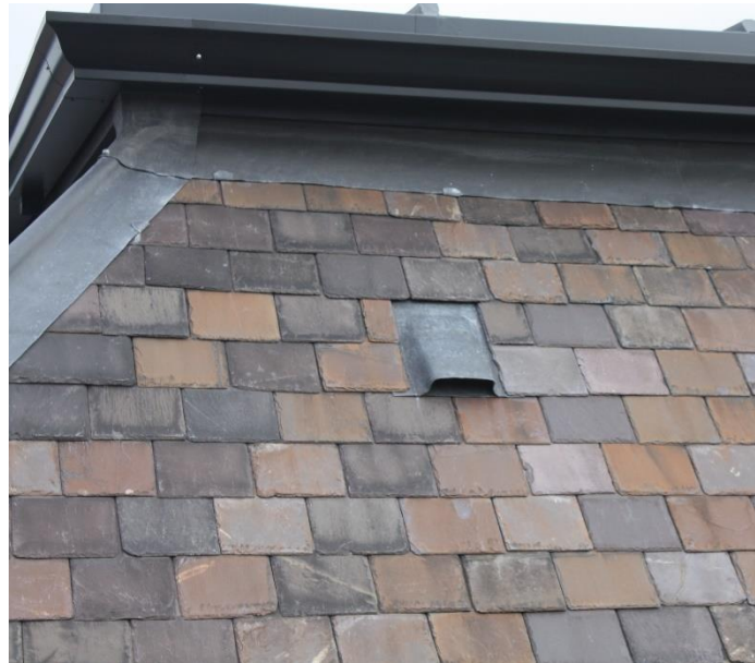
Figure 6.4. Crawl-in access constructed of lead set in slate roof
