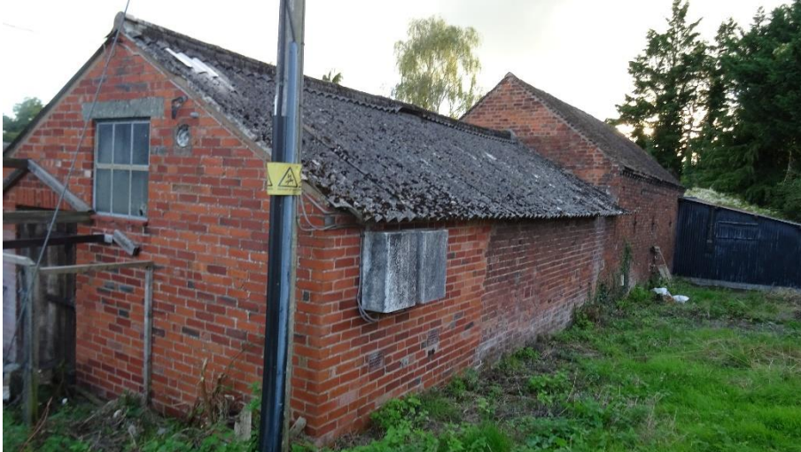
Figure 4.6. Barn 1 from northeast
