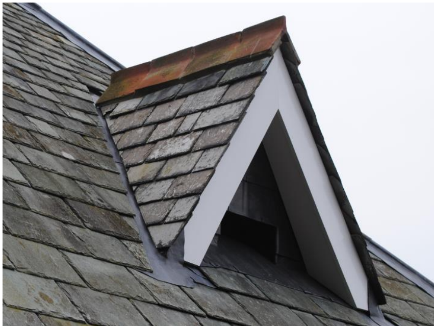
Figure 6.5. Fly-in dormer access external view
