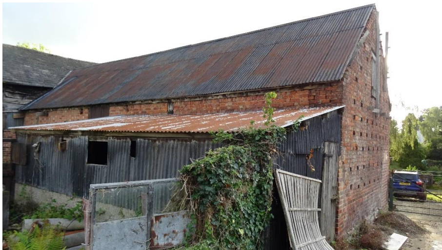
Figure 4.11. Barn 2 north wing
