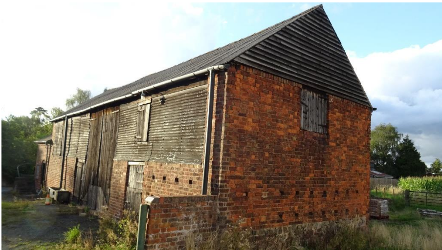
Figure 4.8. Barn 2 from southeast
