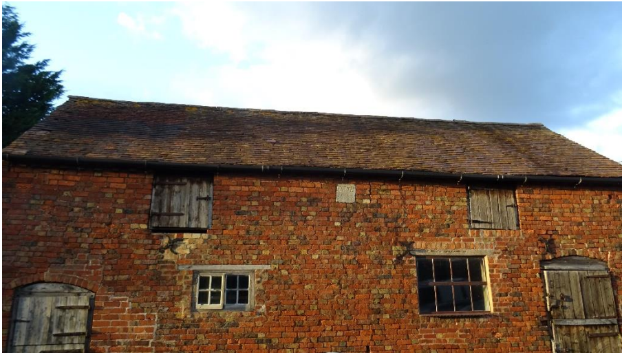
Figure 4.7. Barn 1 from south
