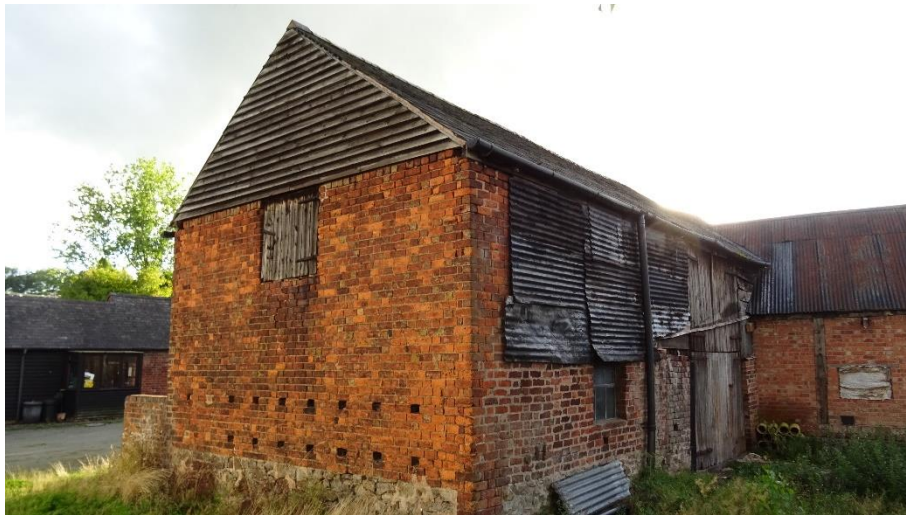
Figure 4.10. Barn 2 east wing
