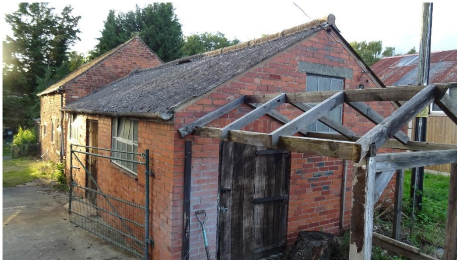
Figure 4.5. Barn 1 from southeast
