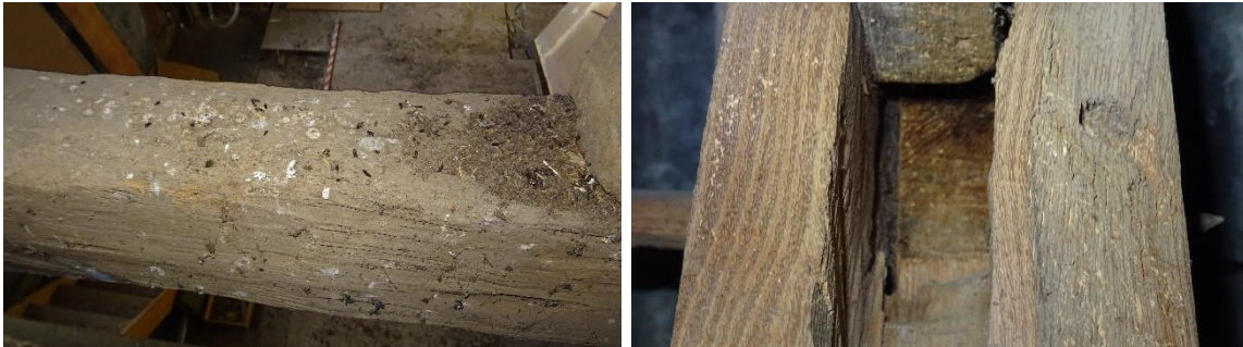
Figure 4.12. Droppings on timber (left) beneath open mortise joint (right)
