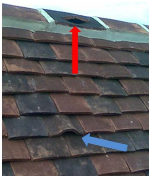
Figure 6.3. Example crawl-in ridge and field tiles
