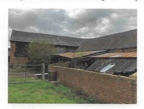
Brickwork to Cow Barn 4 gable apex was fractured above the hatch doors, indicating lack of adequate lintel support and this section will need to be carefully taken down and rebuilt.
