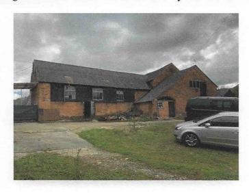
The lower section of wall to Cow Barn 4, adjacent to the ground, was showing signs of damp and weathering, with some perished bricks, but overall was considered to be in reasonable structural condition.
