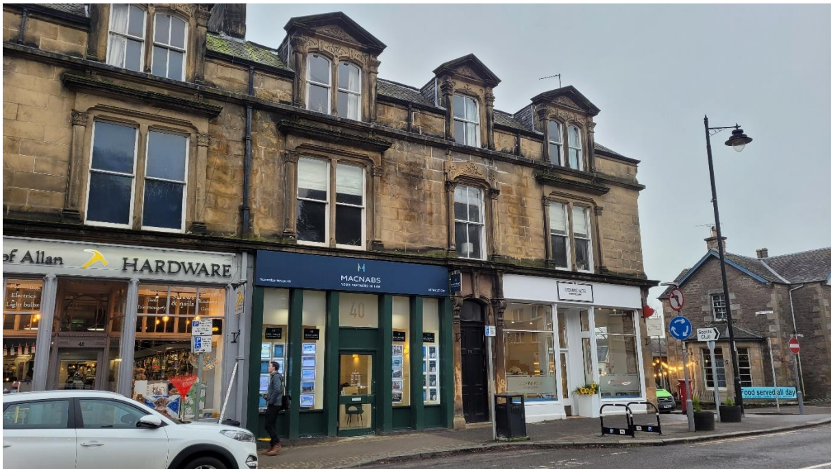
Figure 1. Photo of new signage to the Henderson Street elevation
