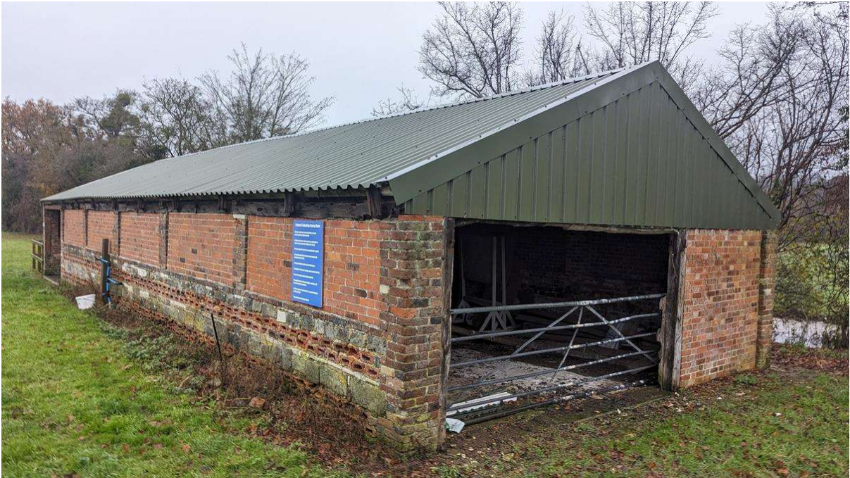
Photo 1 – B1 as viewed from the north-east.
