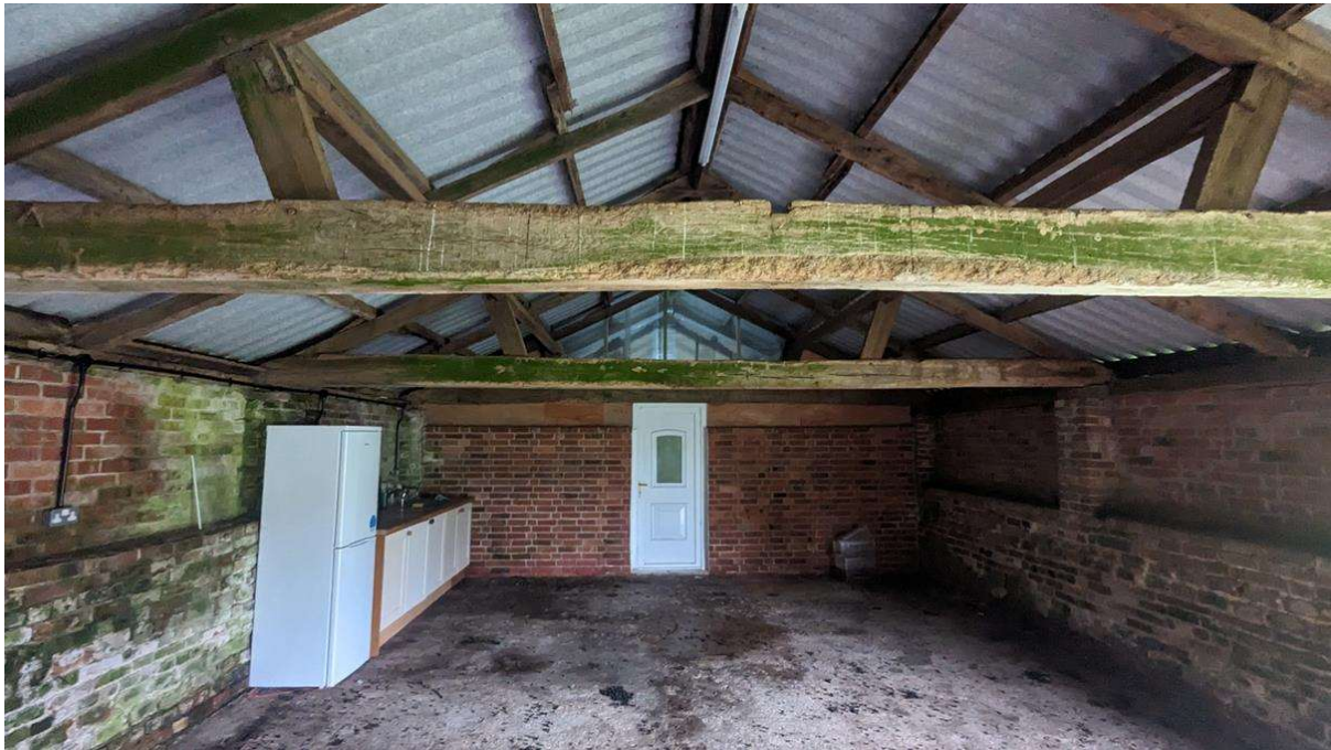
Photo 3 – Looking north to the toilet in B1.
