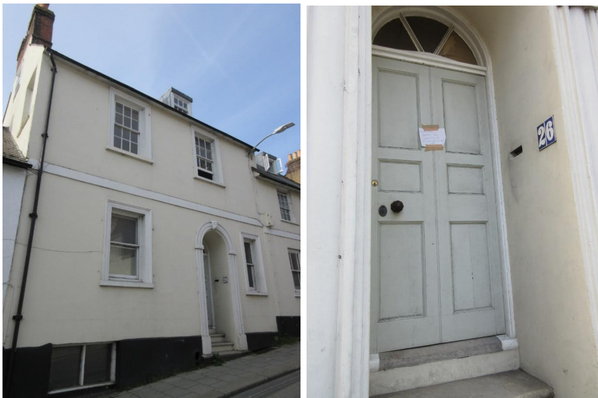
Figure 2 (left): No. 26 Station Street (Grade II).
