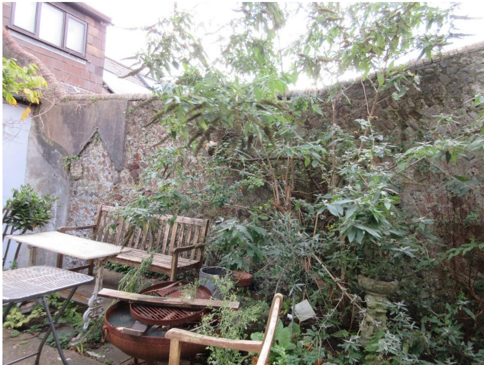
Figure 5: Boundary wall between the garden of the Site and the adjacent site to the south.
