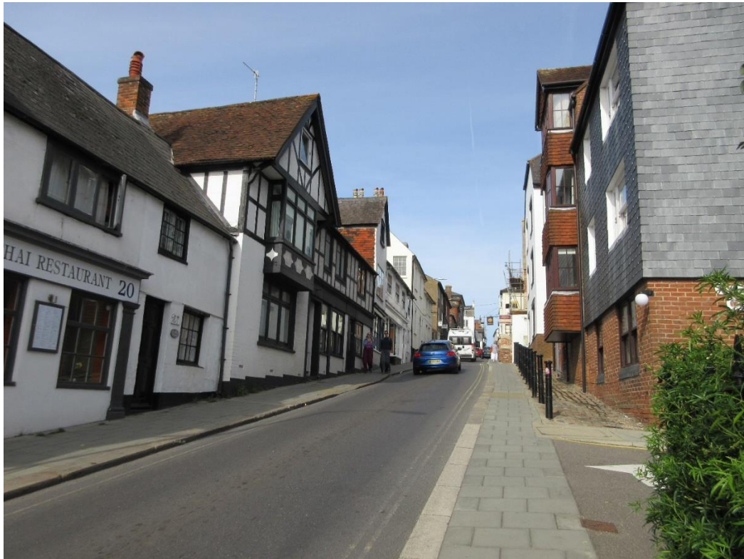
Figure 27: Northern view along Station Street. No.s 19, 20 & 21 (Grade II) can be glimpsed on the left.
