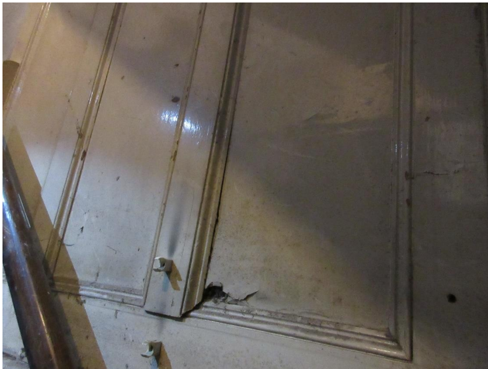
Figure 12: Basement to ground floor – Staircase. Note original timber panelled wall, and timber handrailing.
