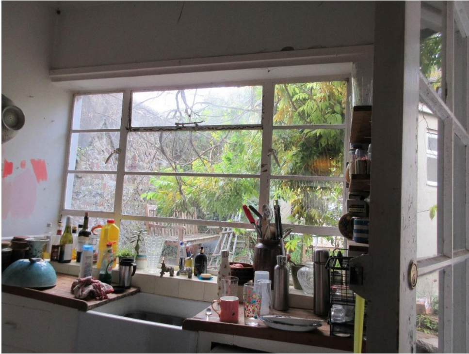
Figure 15: Ground floor – rear extension to Drawing room. Note metal-framed window (likely 1930s-50s).
