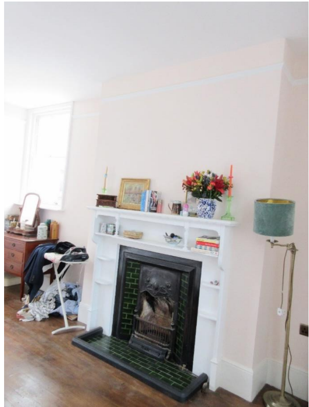
Figure 16 (left): First floor – Westward view looking from the landing towards the bathroom to the rear. Figure 17 (right): First floor – Principal bedroom, to the south. Note original chimney breast and fireplace, and historic skirting and picture railing.
