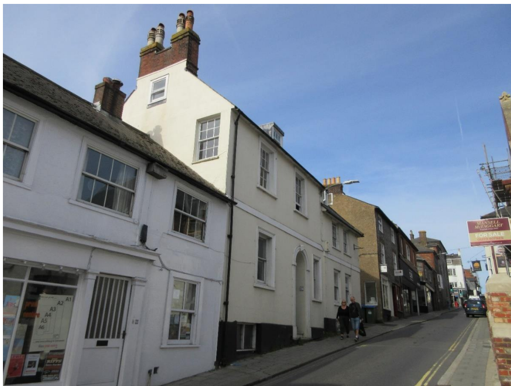
Figure 28: Northern view along Station Street, with no.s 25 and 26 on the left.
