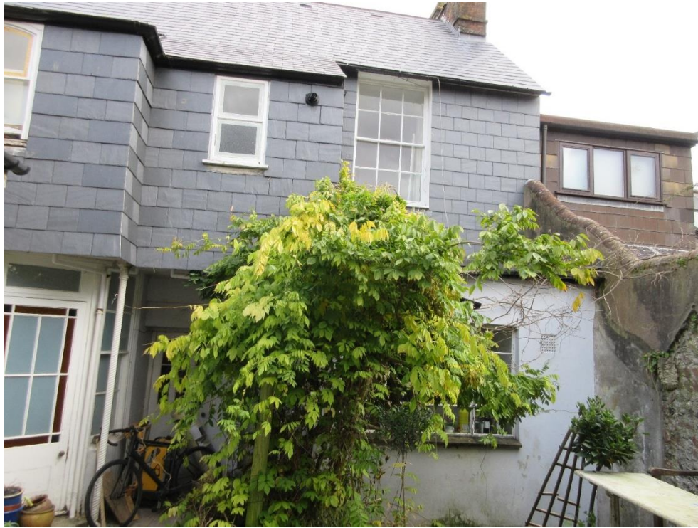
Figure 4: Rear elevation of no. 26. Note single-storey rear extension on the right, and jettied first floor extension on the left.
