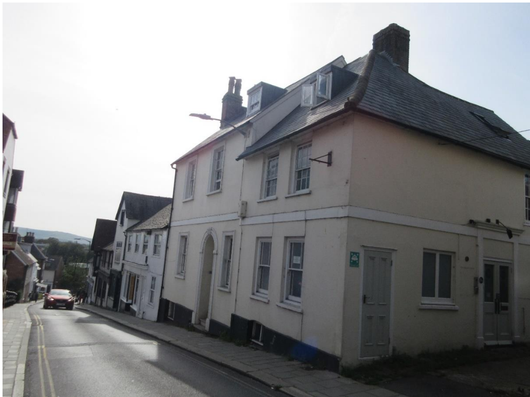
Figure 30: Southern view along Station Street, no.s 26 (Grade II) and 26A (Grade II) on the right.
