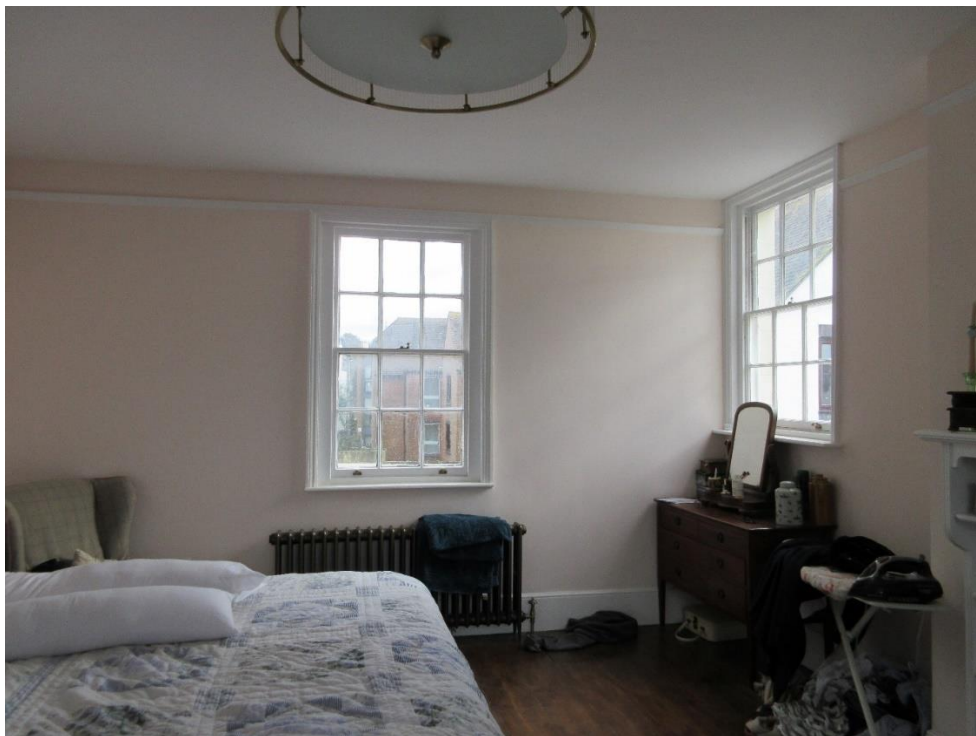
Figure 18: First floor – Principal bedroom, to the south. Note historically correct Georgian-style six-over-six sash windows (including modern window opening on the right), and historic skirting and picture railing.
