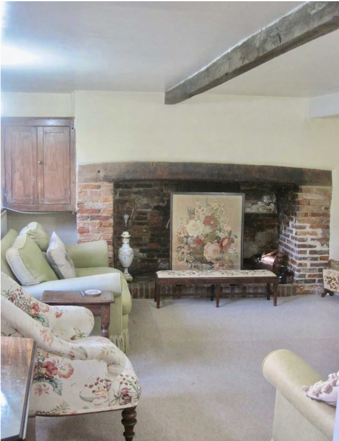
Above: the view looking South of the Living Room showing the original fireplace with 16 th -C. sized hand-made brickwork and authentic beam. The right-hand jamb has been repointed with some replica bricks. This is a feature of 'High Significance' which is extremely important because it dates to the origins of the house, probably 17 th Century. The overhead beam is an original structural timber, more of which survive in the attic.
