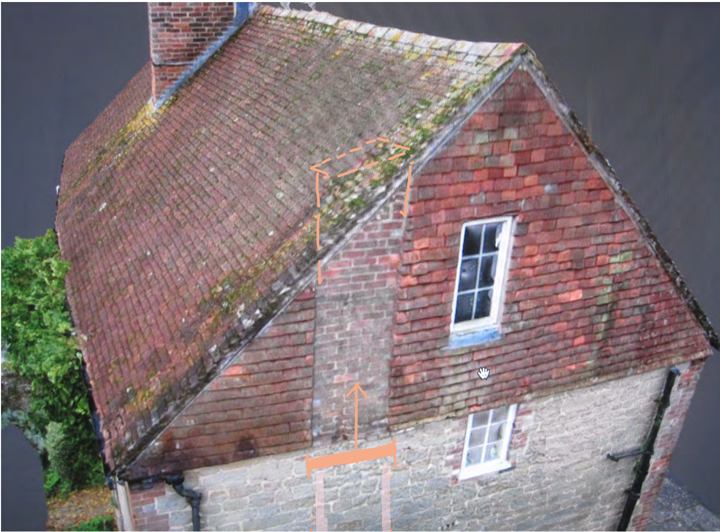
6.2.3. Above: the drone photograph of the north end gable of 330 Grove Street. This clearly shows the ‘ghosting’ where there appears to have been an earlier chimneystack behind what is currently the front entrance door. This also appears in the thicker brickwork of the Ground Floor plan here, and also corresponds to a similar chimneystack for the Kitchen at No.331, although this survives at the rear where one would normally expect it to be located.
