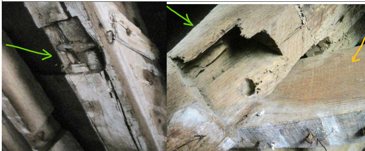
Above: both pictures show ‘ghosts’ of missing lathe & plaster (white marks) + nails . This shows that the attic was altered, so it was likely used as a bedroom at a later date.
