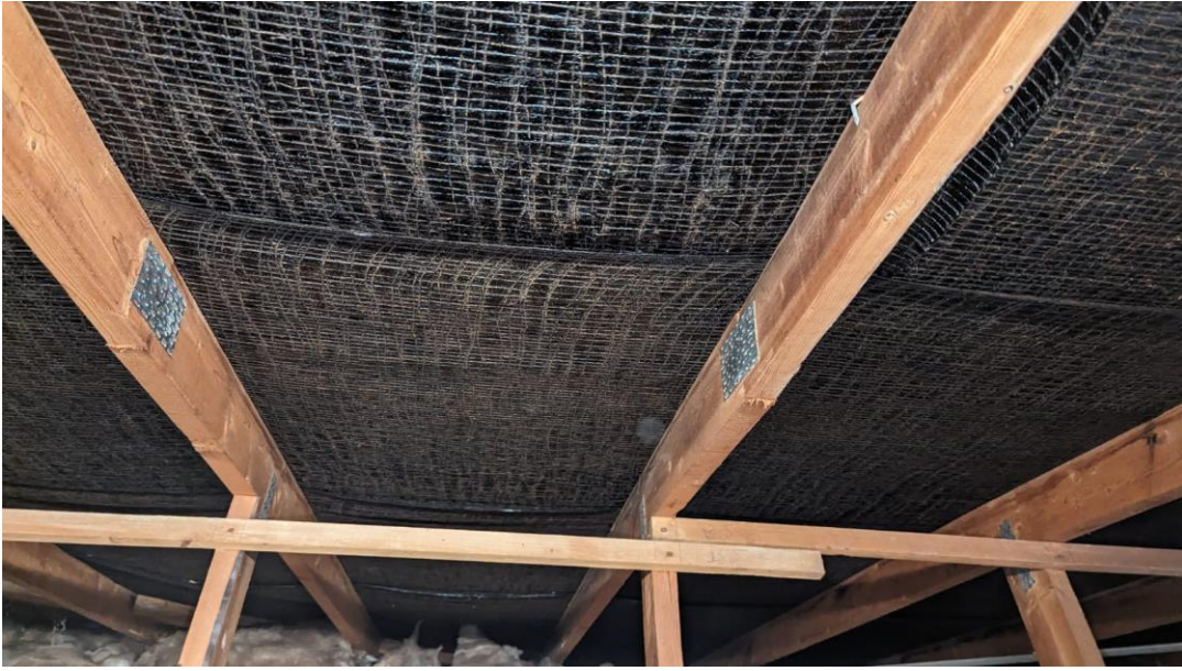
Photo 3 – Internal loft void
