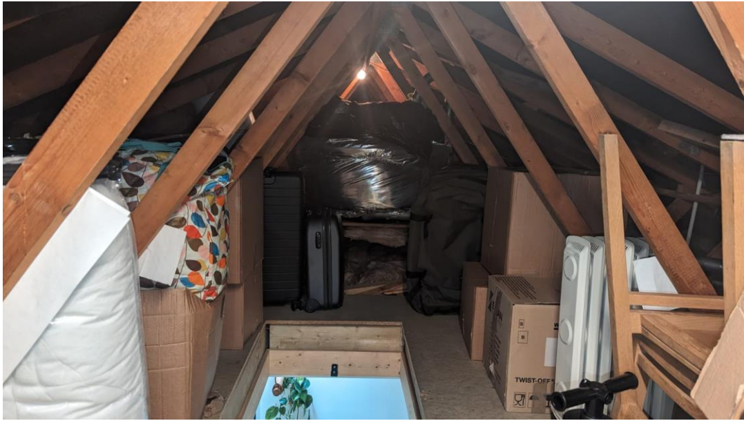
Photo 1 – Internal loft void
