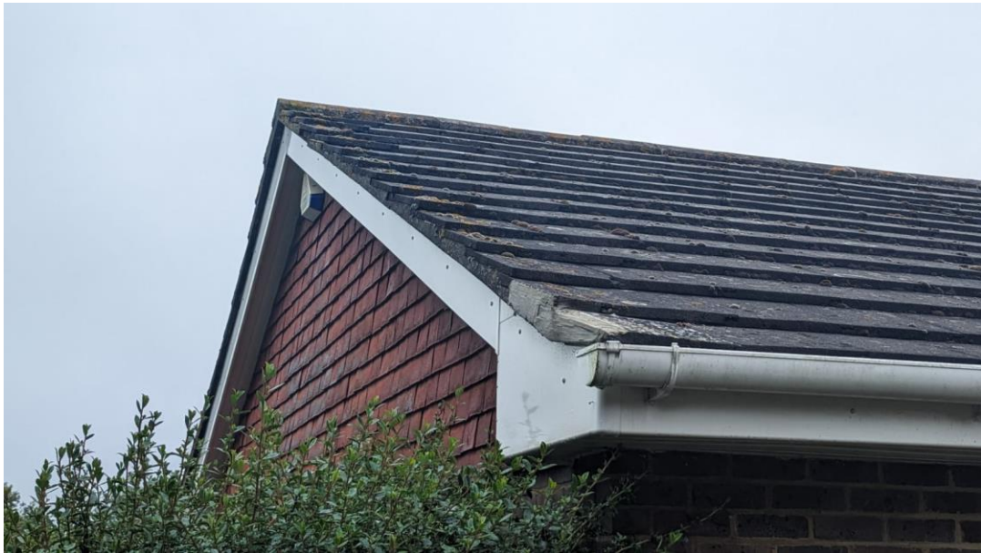
Photo 7 – Hanging tiles on gable
