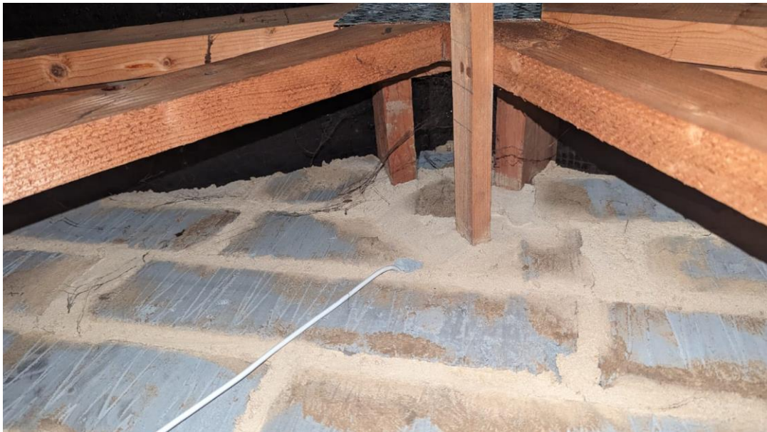
Photo 2 – Internal loft void
