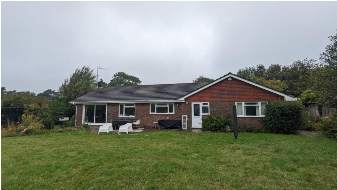
Photo 6 – South facing elevation
