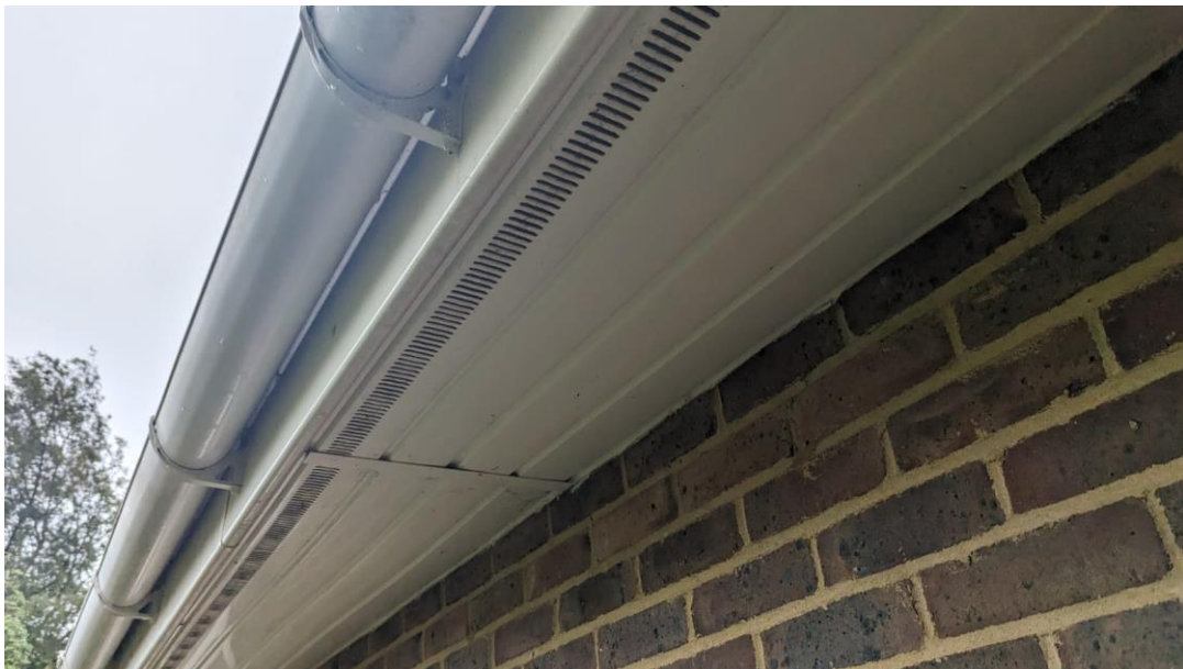
Photo 8 – Soffit and fascia made of modern uPVC
