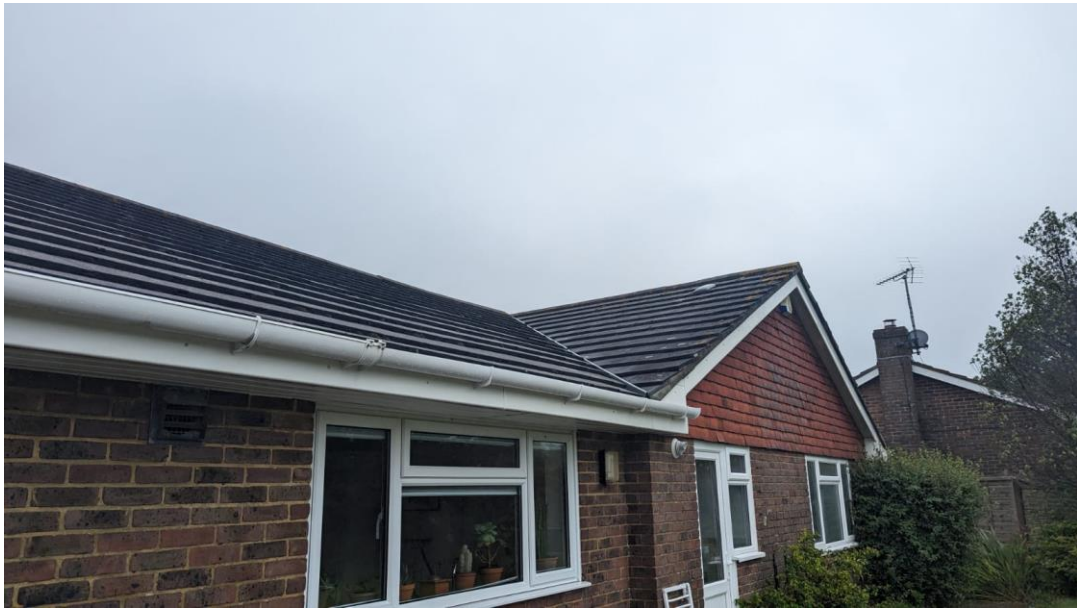
Photo 9 – Concrete slab roof tiles and hanging tiles on gable
