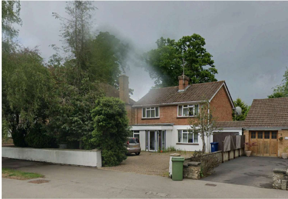
Figure 6: The existing site from the front
