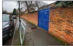
Existing gate to be replaced
