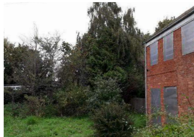
View of Hostel building looking West
