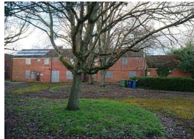
Existing Hostel building South elevation
