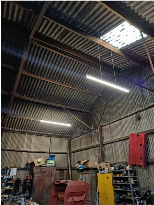
Photo 4: TN7 - interior typical shed
