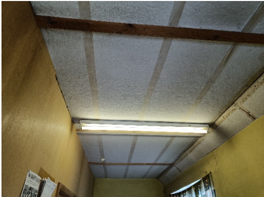
Photo 2: ceiling inside low brick building
