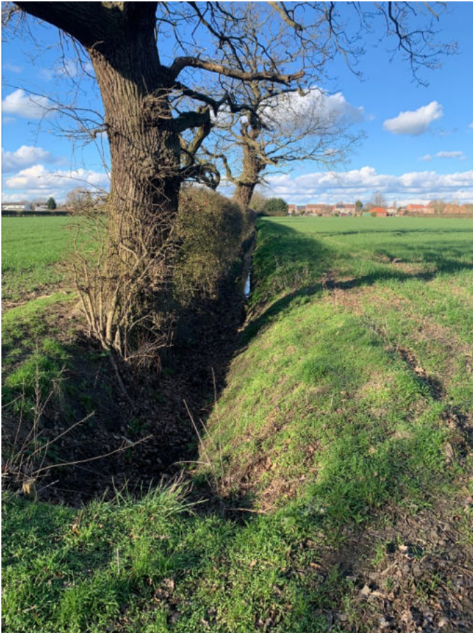
Figure 9 – Intakefield Drain in centre of site. View N.
