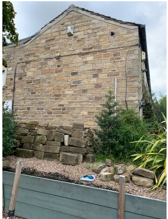
Photograph 4- View looking north-west (Side Elevation)
