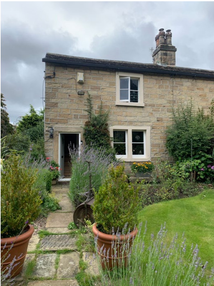
Photograph 1- View looking south-west (Front Elevation)
