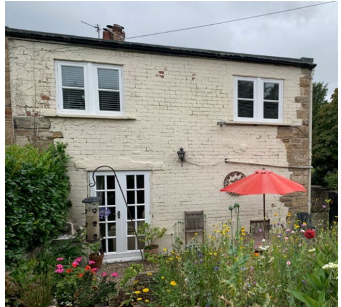
Photograph 2- View looking north-east (Rear Elevation)
