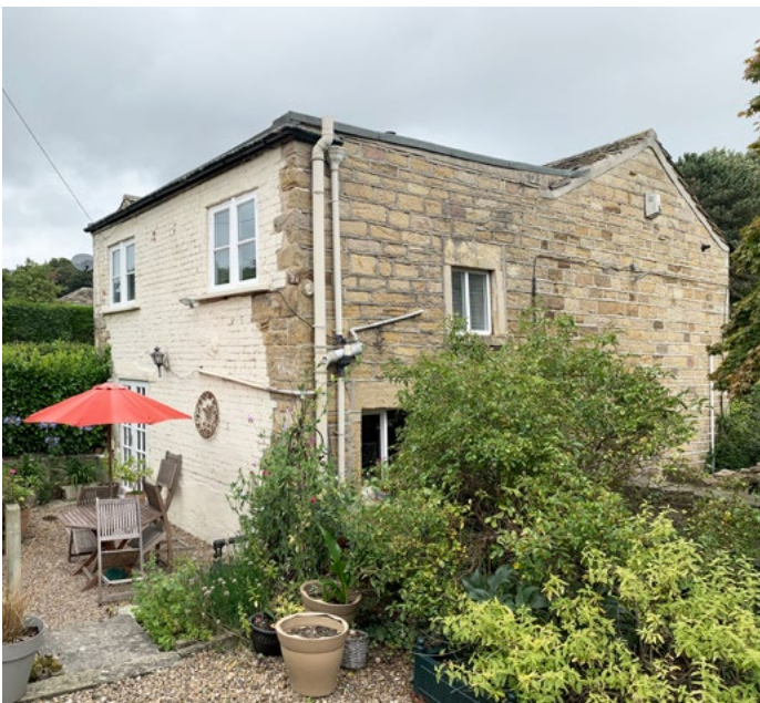
Photograph 3- View looking north (Rear/ Side Elevation)
