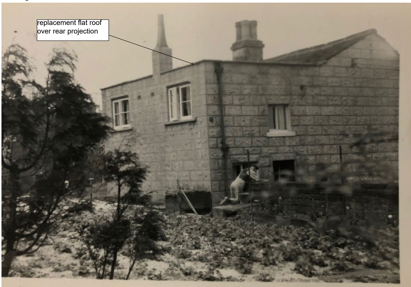
Photograph taken c1920 looking north towards the side and rear elevations / projection of Gardeners Cottage, 19 Hall Lane
