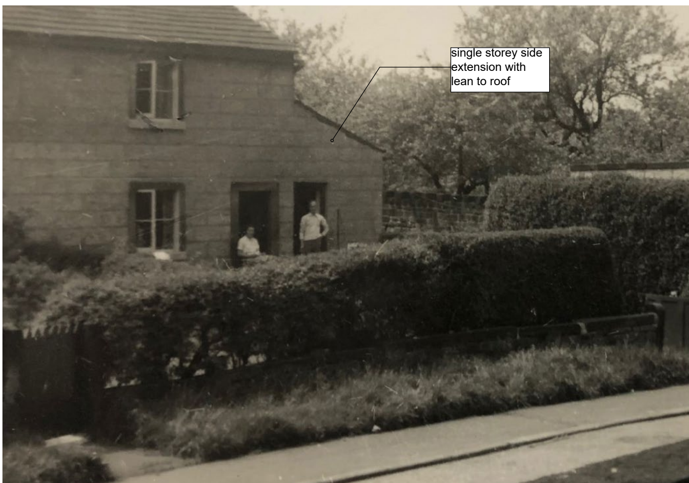
Photograph taken c1920 looking east towards the principal entrance of the adjoining Cottage at number 21 Hall Lane
