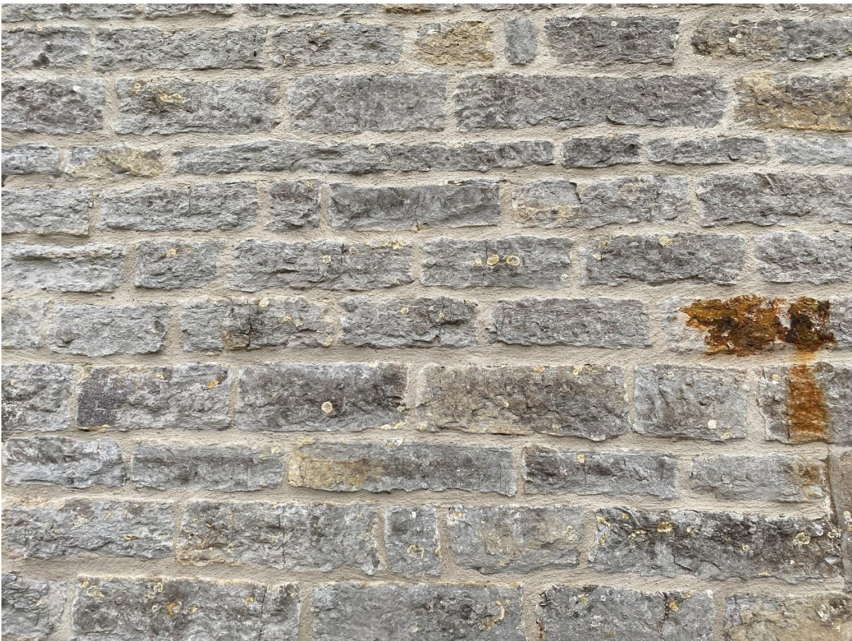
Image 2 – Detail photograph of wall to Farmhouse showing repointed mortar.
