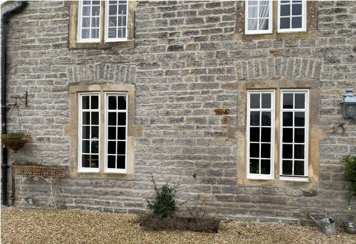
Image 1 – Photograph of wall to Farmhouse showing example of repointed mortar.
