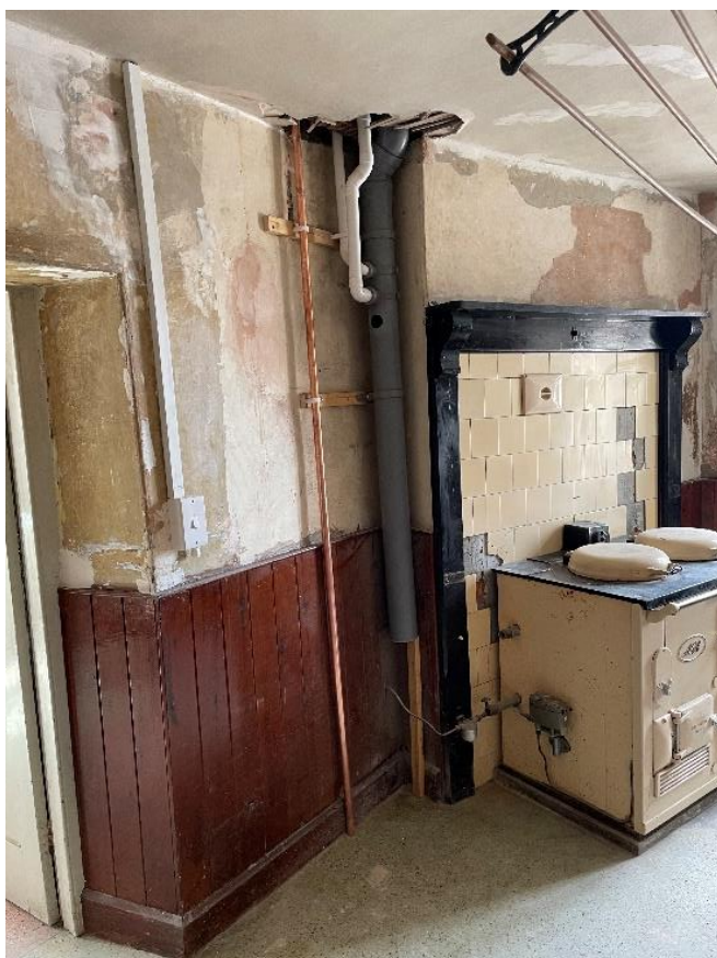
Image 4 – Fireplace to ground floor Snug (GF5) prior to renovation work.
