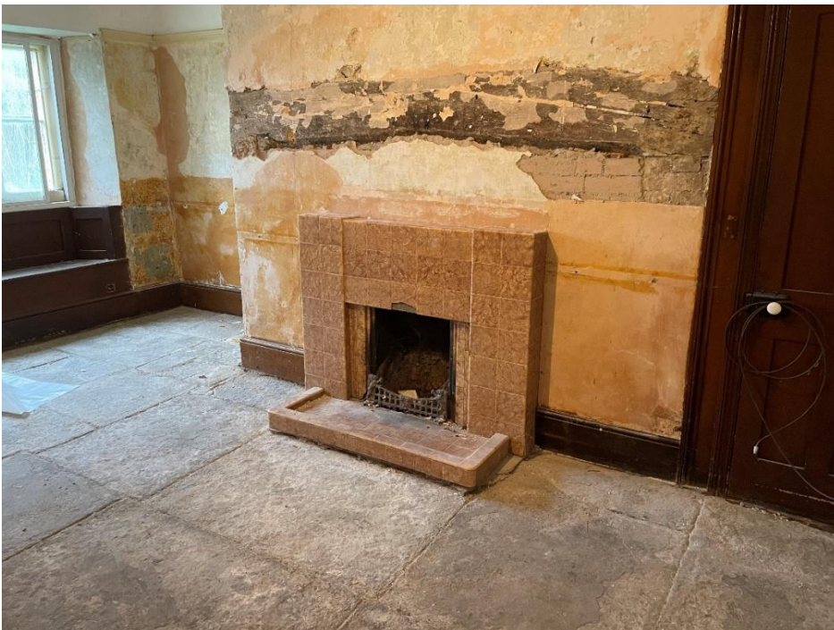
Image 2 – Fireplace to ground floor Dining Room (GF1) prior to renovation work.
