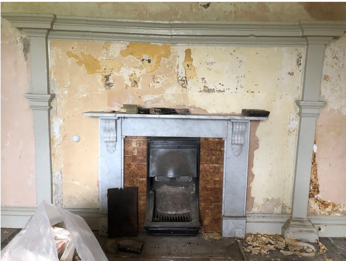
Image 6 – Fireplace to ground floor Living Room (GF2) prior to renovation work.
