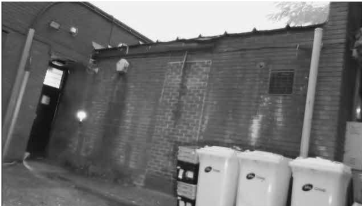
Plate 1: View of the north western aspect taken by surveyor ET at on 29/08/2023.
