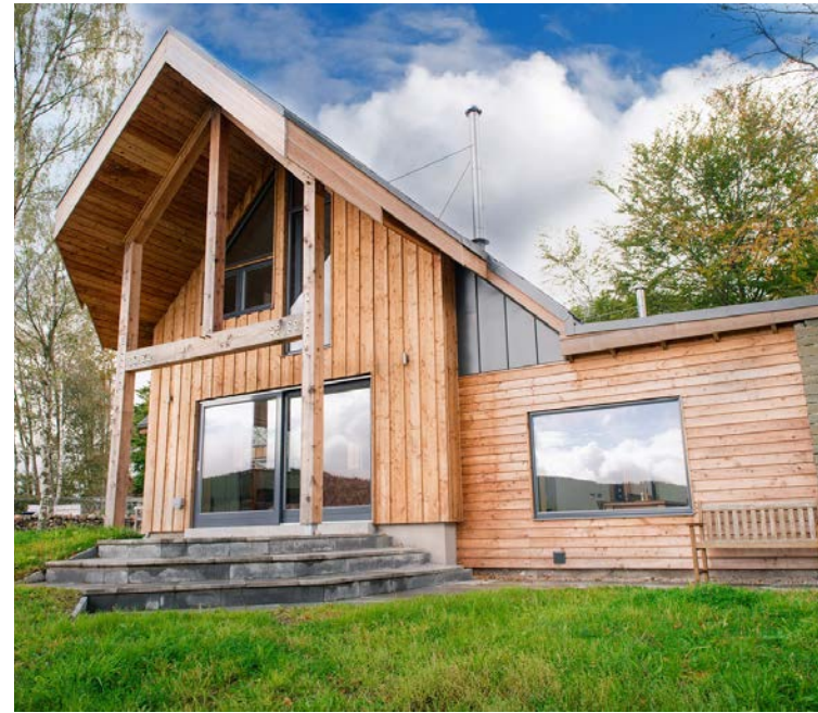
Timber and steel post
