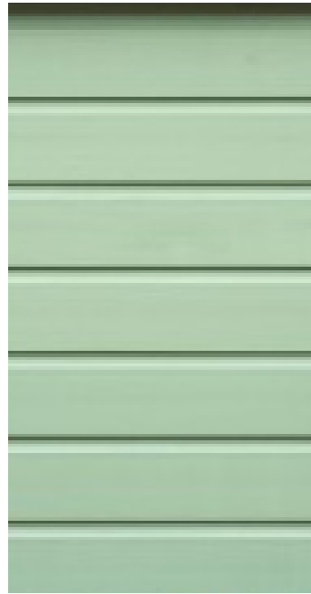
Painted Timber Cladding
