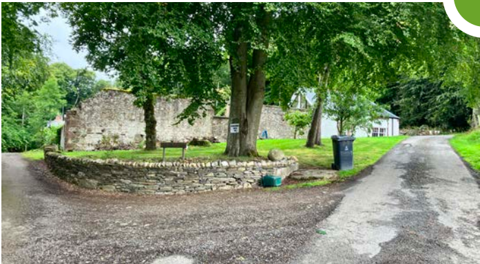
Stone Wall to North of Tennis Court Retaining Old Road Above
