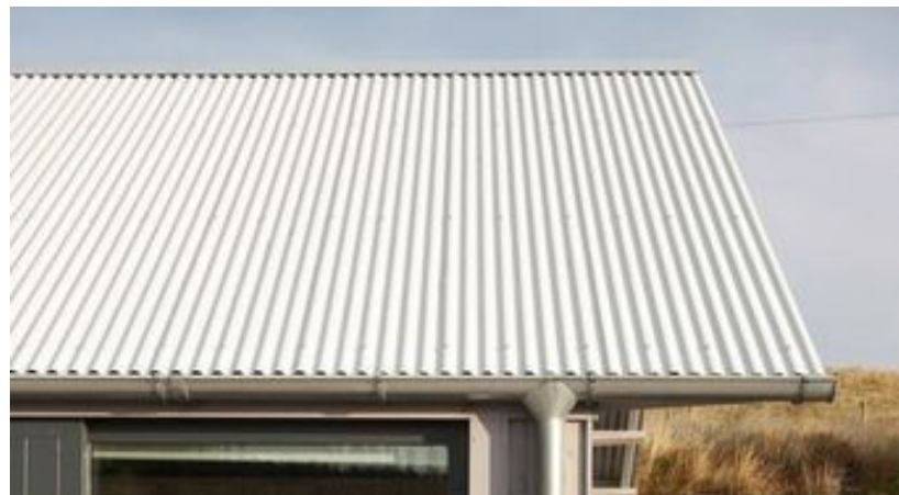
Corrugated Metal Roofing
