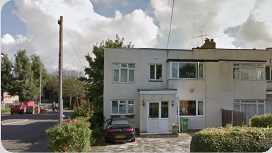
192 Rectory Road, Basildon, Essex SS13 2AN - Front View
