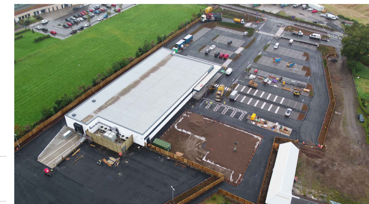
ROOF EXAMPLE (ALDI CRIEFF) - KINGSPAN "TOPDECK" KS1000/91/TD/ECOSAFE/LPCB COMPOSITE MEMBRANE COVERED ROOF PANELS, COLOUR: RAL 7046 (TELEGREY 2)
