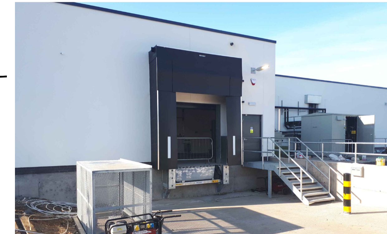
WHITE RENDER AND LOADING DOCK EXAMPLE (ALDI CRIEFF) - THROUGH-COLOURED WETHERBY RENDER SYSTEM
