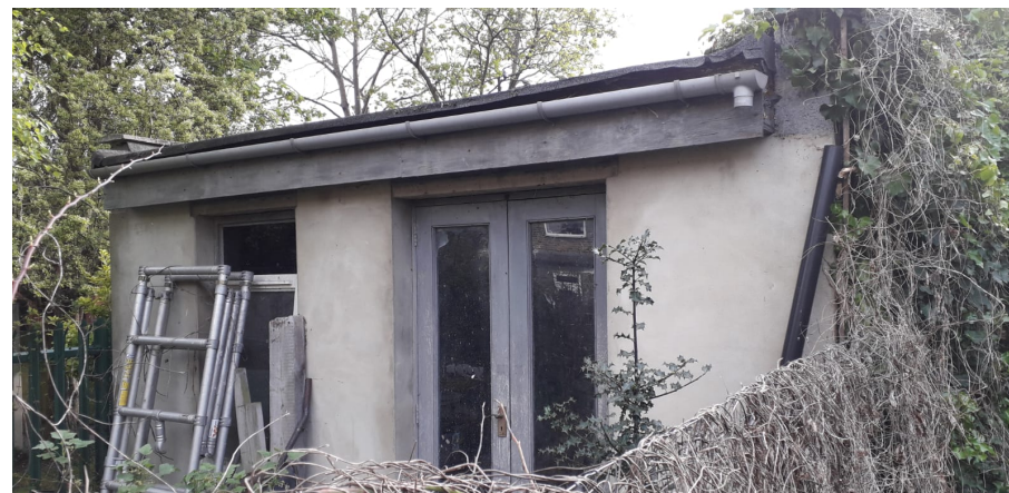
EXISTING NEIGHBOUR SHED TO LEFT HAND SIDE
