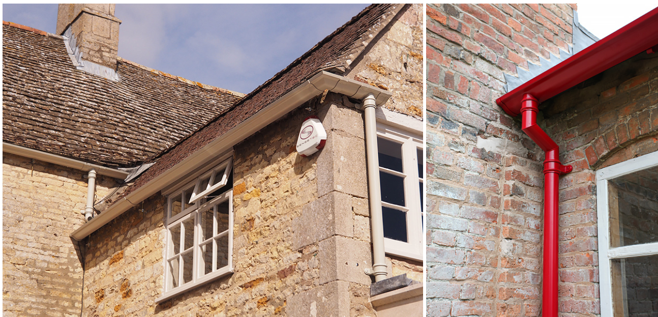
Images 04 & 05 – Examples of new cast aluminium guttering & downpipes in the traditional OGEE style
