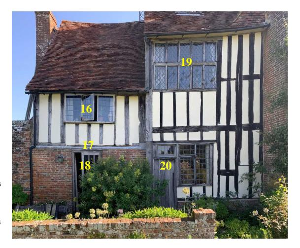
**Item Number 18 Condition** Poor, the door leaf has racked and door cill is degraded, glazing bars in poor condition
