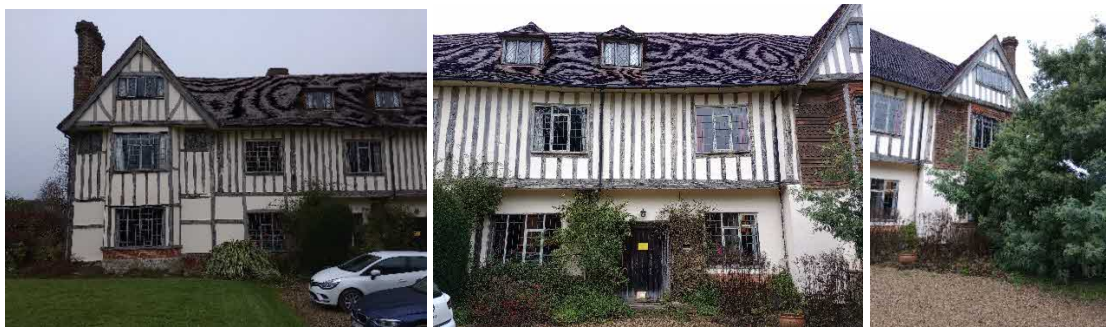
Front (South-east) elevation: South end centre East end
