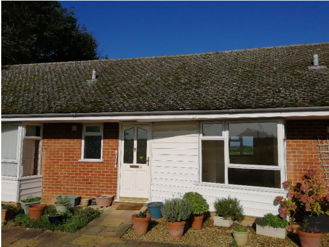
Photograph 5: Closer view of south elevation of far west cottages (Cottage 2)
