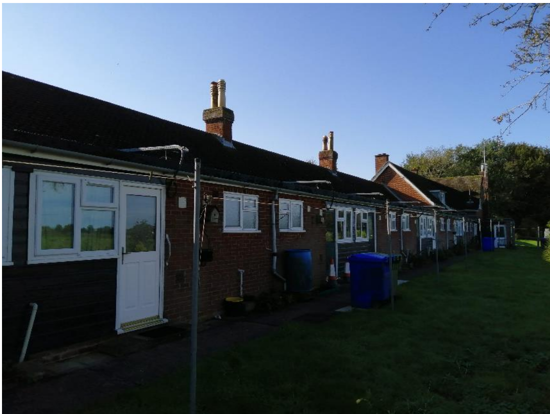
Photograph 2: North elevations of the cottages
