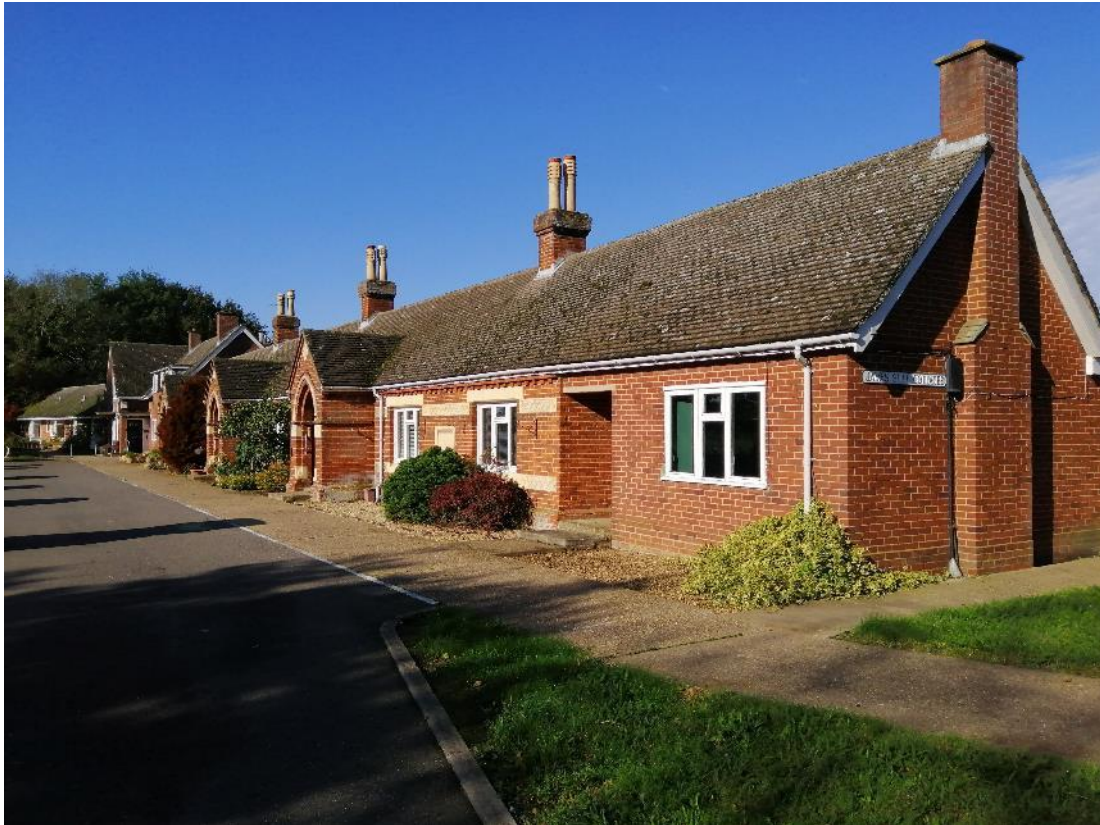
Photograph 1: South and east (left – right) elevations of the cottages
