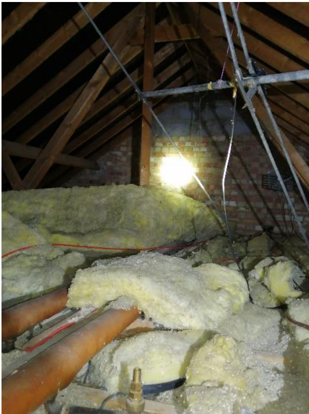
Photograph 10: Example of inspected loft space
