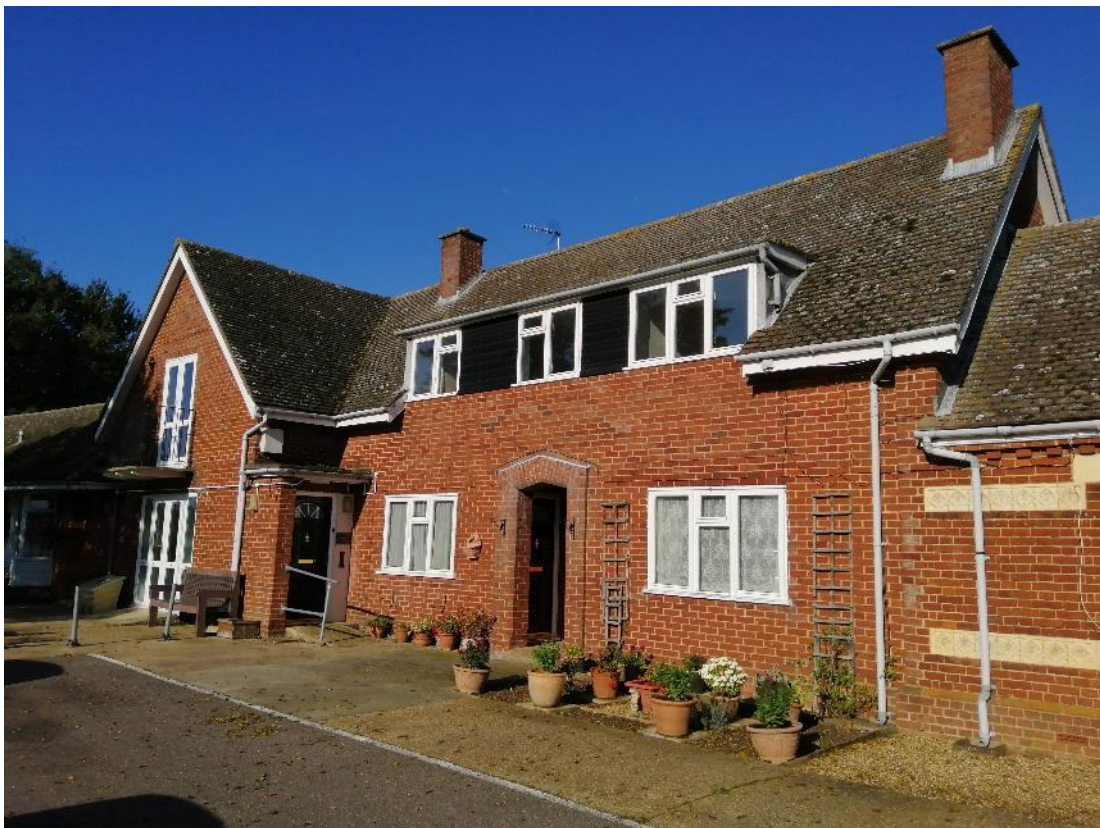
Photograph 4: South elevation of the two-storey Cottages 5, 6 and 7 (left – right)
