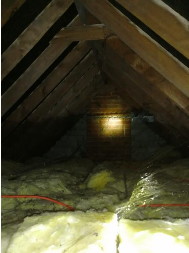
Photograph 9: Example of inspected loft space
