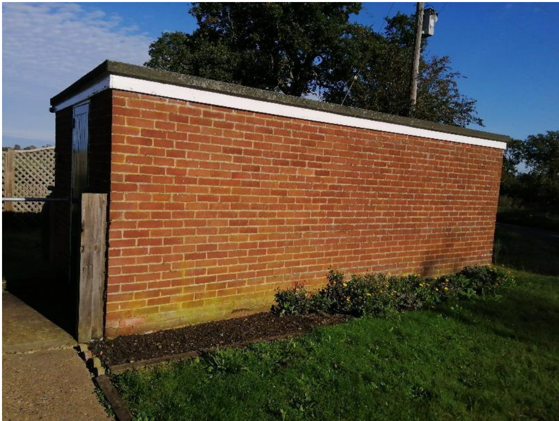
Photograph 8: South and east (left – right) elevations of detached outbuilding
