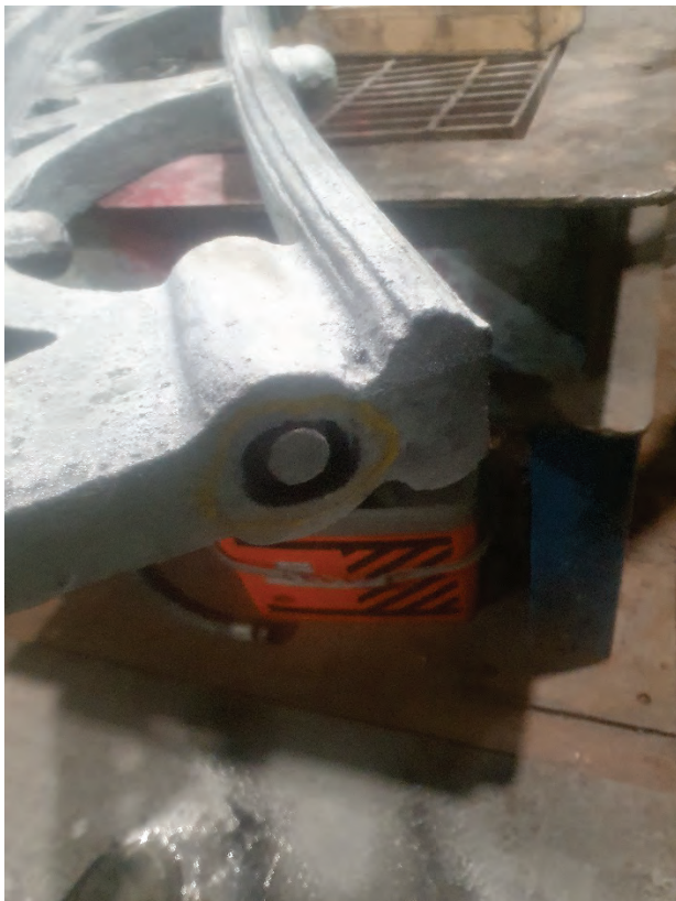
Photograph 10, seized bolt to corbel / spandrel connection. Bolt could not be readily removed without heat.
