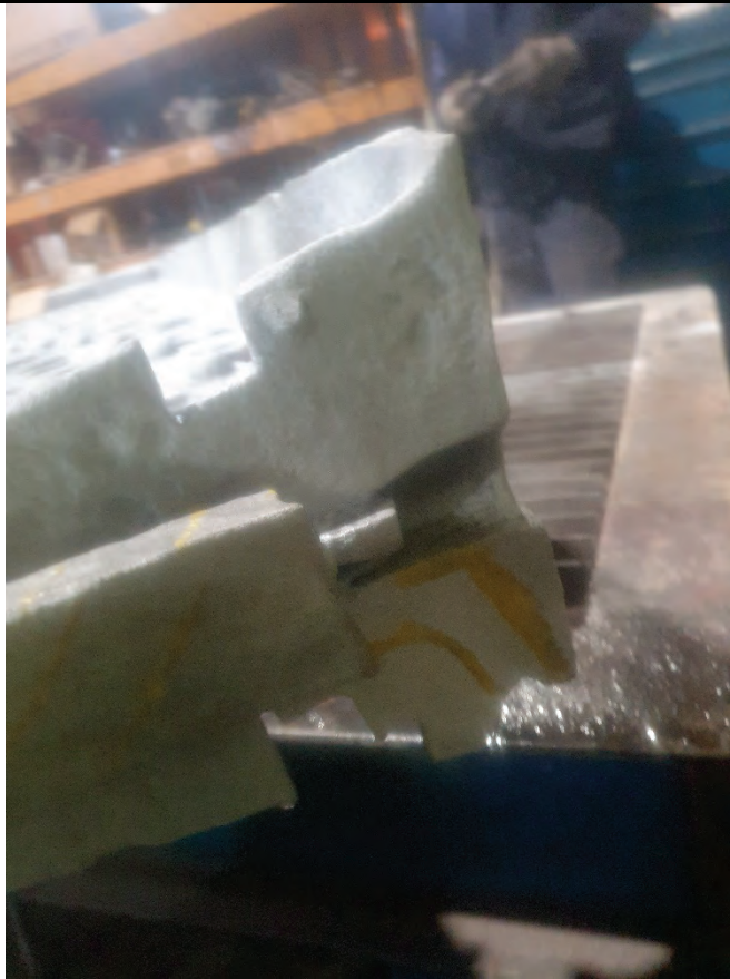
Photograph 7 indicating fracture to keystone top.
