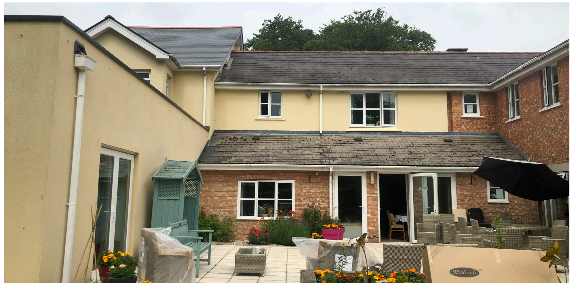
Photo showing the existing Patio area where the Lounge Extension is to be built
