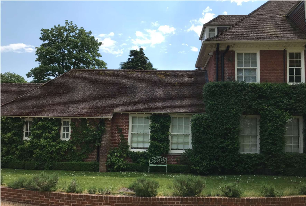
Figure 4: Part view of existing single storey extension
