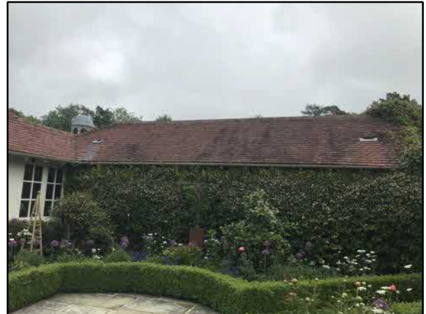
Image 2: A view of the western elevation of the pool house.
