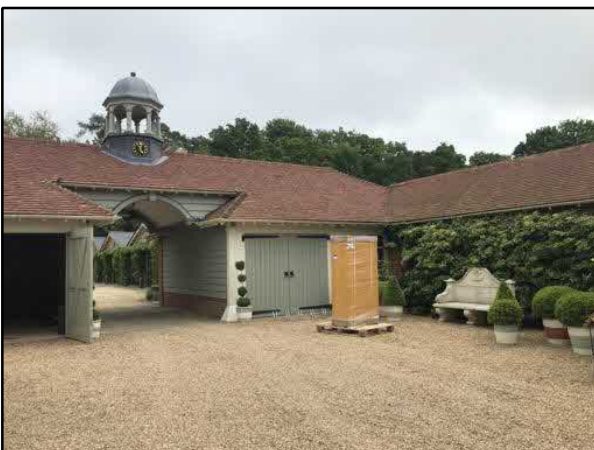
Image 5: A view of the western elevation of the northern wing comprising the washroom, archway and garage
