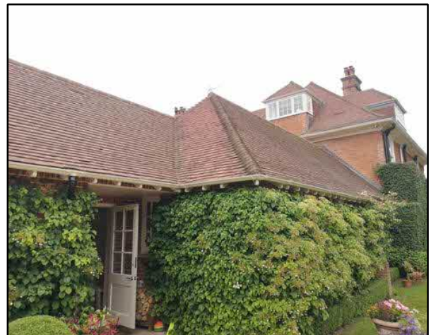
Image 4: A view of the northern elevation of the extension.
