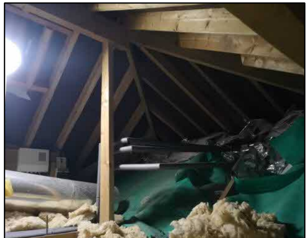
Image 10: A view inside the small void present in the northern wing.
