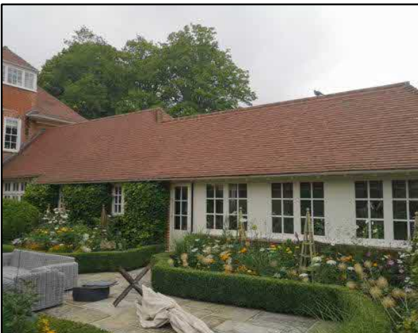
Image 3: A view of the southern elevation of the extension.
