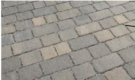
Front Driveway Tegular Block
