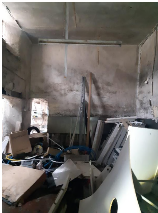
Figure 5: Internal area of the single storey building.
