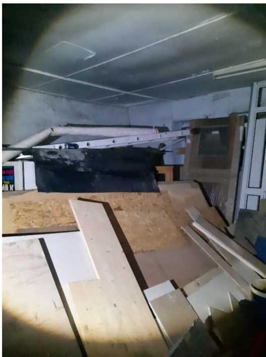
Figure 6: Internal area of the two-storey building to the south (first floor)
