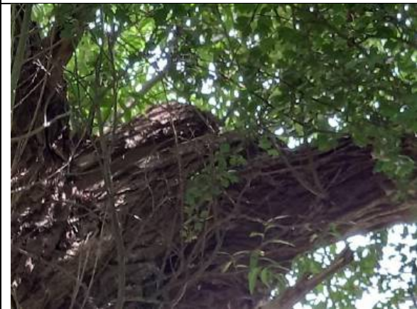
Photograph 9: White willow in G6 with split in branch
