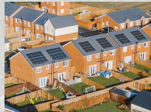
PV panels on a completed scheme by Breck Homes
