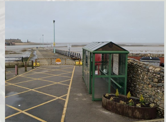
Knott End Ferry Slipway
