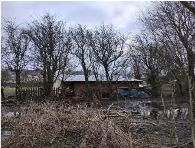
Figure 9 – Displays a section of the northeastern site boundary where a horse stable is located.
