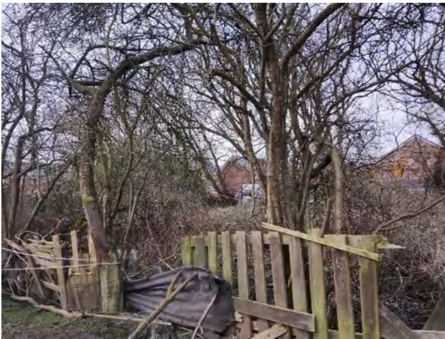
Figure 27 – Displays the northwestern site corner which has been segregated using wooden panels and corrugated metal sheets.
