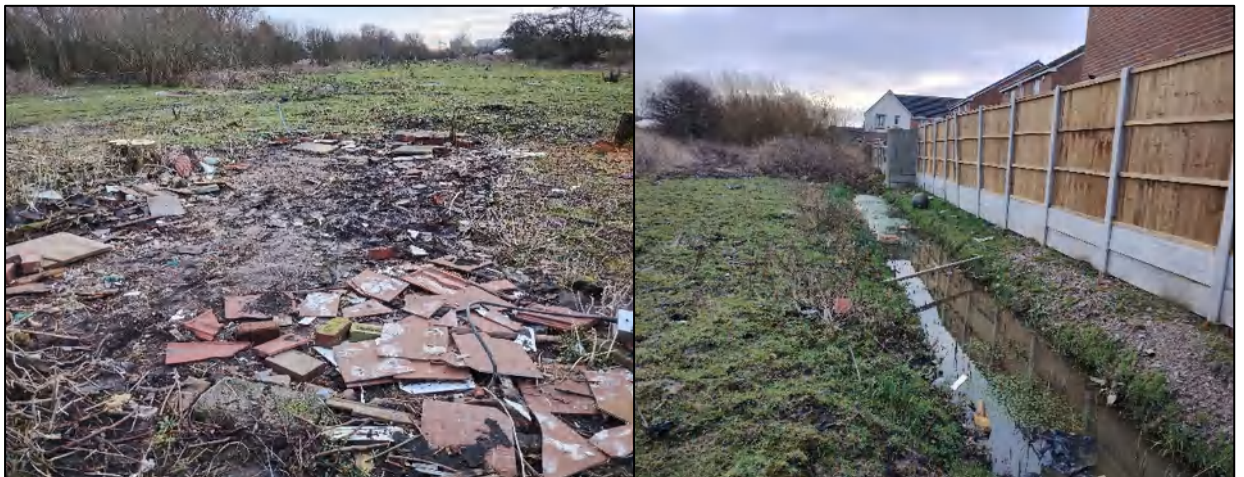
Figure 7: Photograph showing evidence of fly tipping in the northern site section (left) and the debris observed in the drainage ditch on the western site boundary (right).
